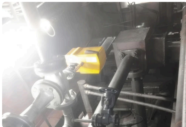
The motorised Jetomat® (Baelz 590) DN50 at the vulcanising press.
